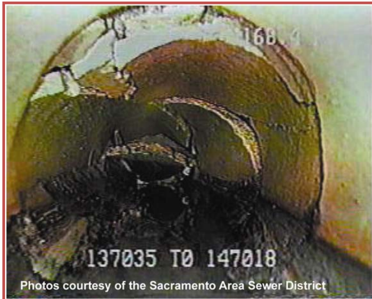
Cracked Pipes
