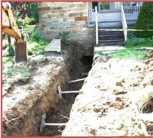
Photo of a trench repair
